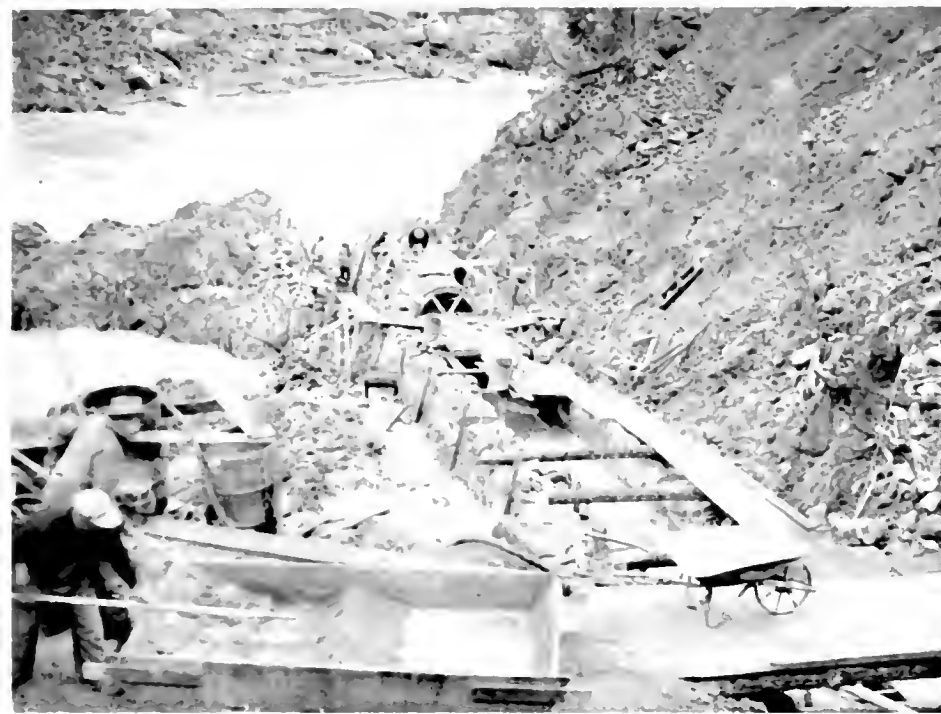
Fig. 52. Left—Masonry arch culvert under construction. Right—Same culvert unequally loaded by end-dumped material on one side (material to be rehandled to a lower level for compaction).
